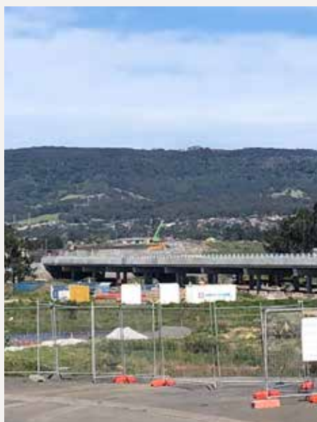
🚧 Albion Park Bypass is expected to open in 2022.
