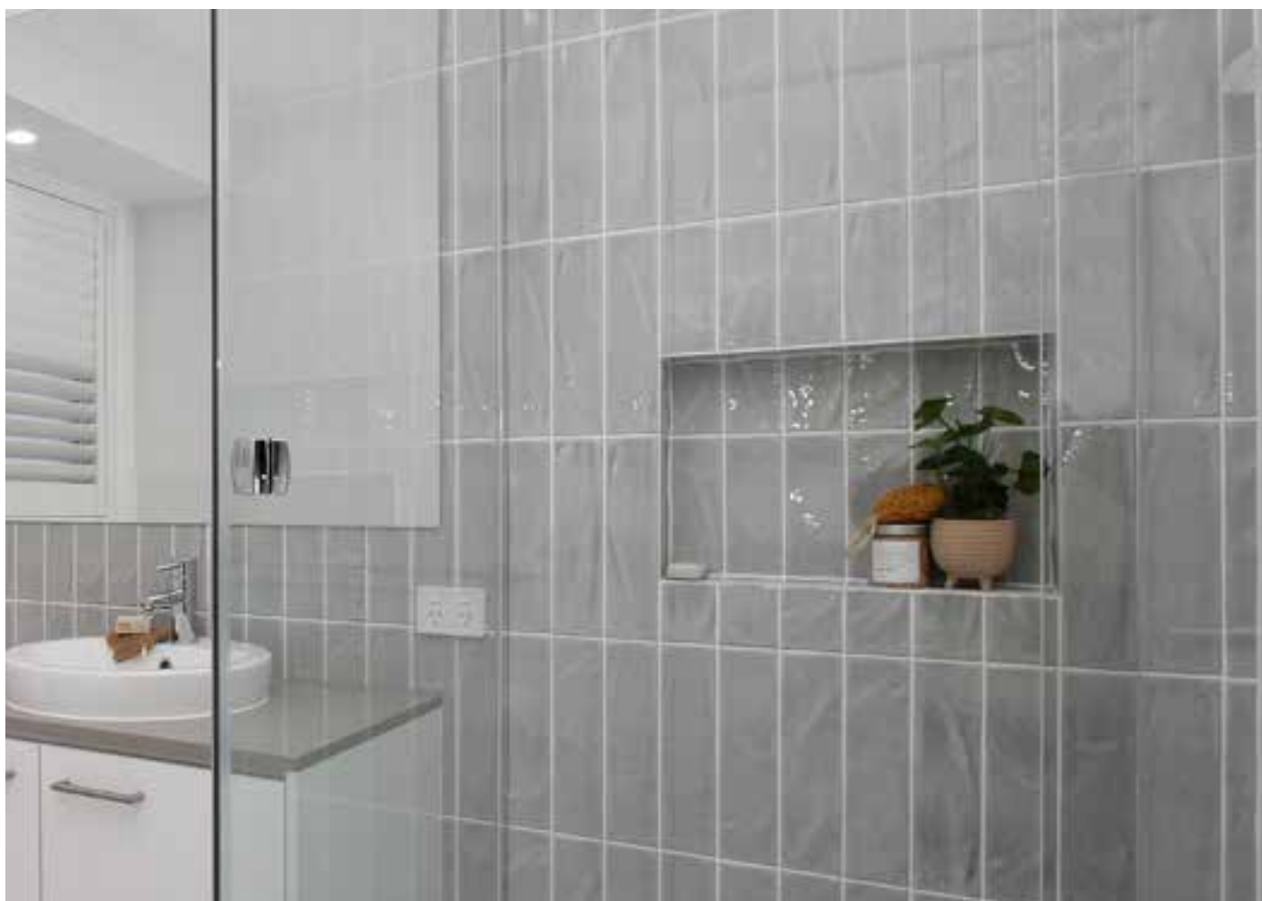
Shower Niche to Ensuite and Main Bathroom
