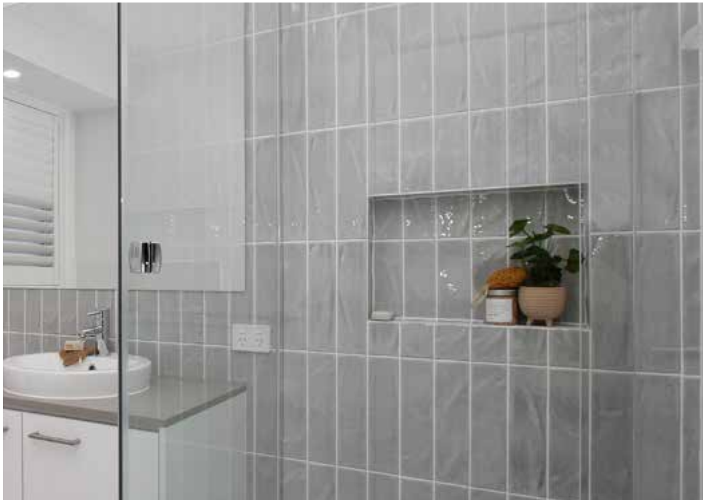
Shower Niche to Ensuite and Main Bathroom
