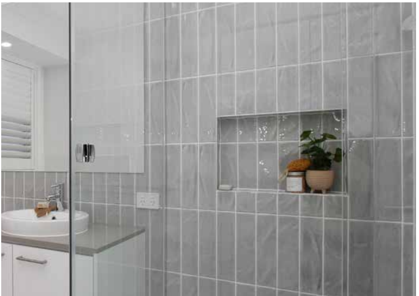
Shower Niche to Ensuite and Main Bathroom
